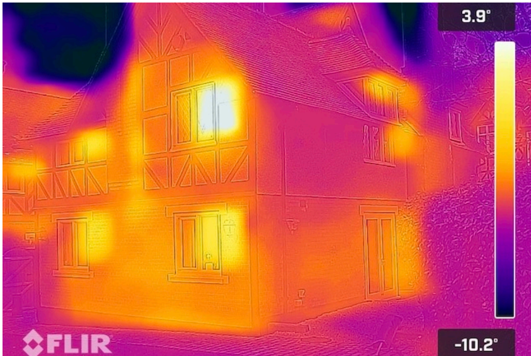
THERMAL IMAGE OF A GRADE 2 LISTED HOME “HEATING THE SKY” DURING VISIT FROM BEAST FROM THE EAST 2 - FEB 2021
